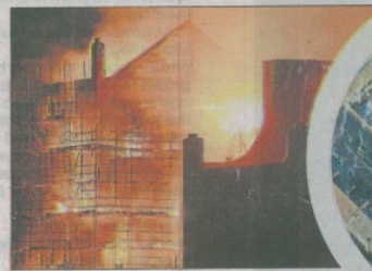
A second damaging fire rips through Glasgow School of Art in June 2018, and inset, overhead view of stricken Mackintosh building
